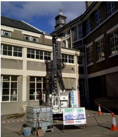
ERS was requested to investigate a high school site as part of re-development proposals for construction of new school premises. The purpose of the investigation was to determine potential foundation solutions and to assess any potential chemical contamination and ground gas issues.
