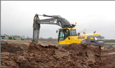
Soil Stabilisation has many attractions in today's construction market. Cost and environmental benefits figure largely in the appeal of the soil modification process which enables granular and cohesive soils to be upgraded by the in-situ mixing of binders with the host material. ERS utilises a range of techniques to convert previously unworkable, weak or contaminated soil into durable, cost effective construction material.
