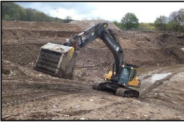
**Soil separation is a key part of any ex-situ soil remediation scheme. The process entails segregation of impacted soils from non-impacted soils, and soils with differing levels or nature of impact from each other. This starts with the excavation process, identifying and separating the various strata 'at source'. Further separation can be used to remove boulders, concrete etc that might not need the same level or type of treatment as the impacted soil.**
